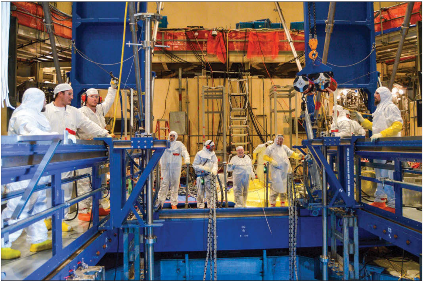
Water jet peening crews from Mitsubishi Nuclear Energy Systems and AZZ/WSI observe the refuel pool from above as both peening tools perform the process inside the reactor vessel. (Photos: Scott Bolley/Wolf Creek Nuclear Operating Corporation)
