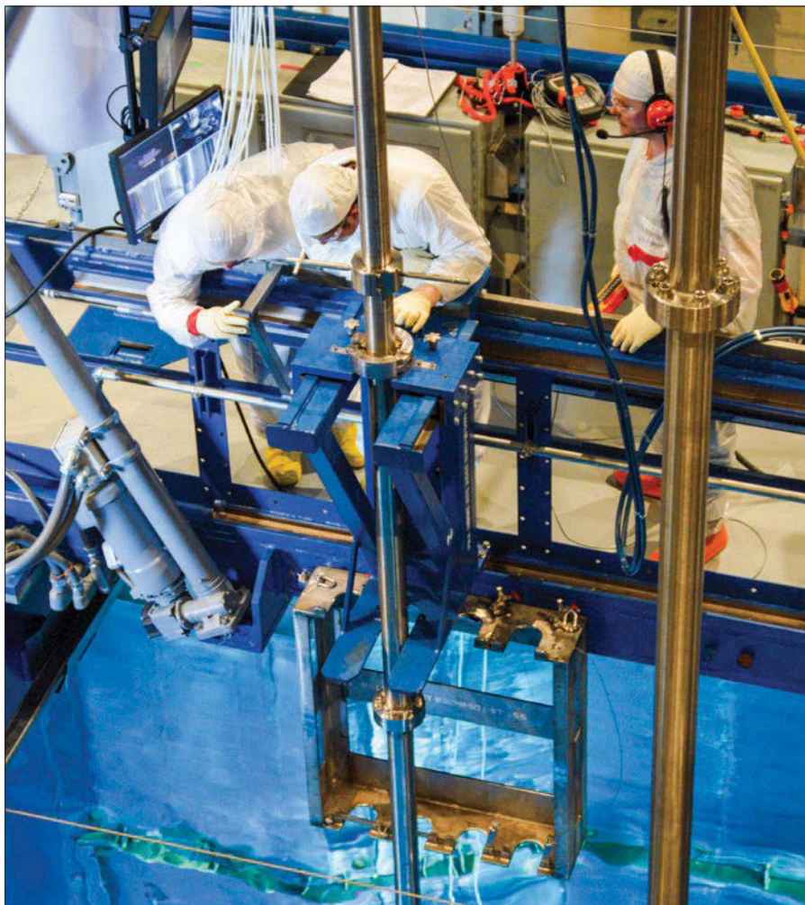
Workers lower the peening tools into the reactor vessel via metal extension rods, positioning them to begin peening a particular area.
